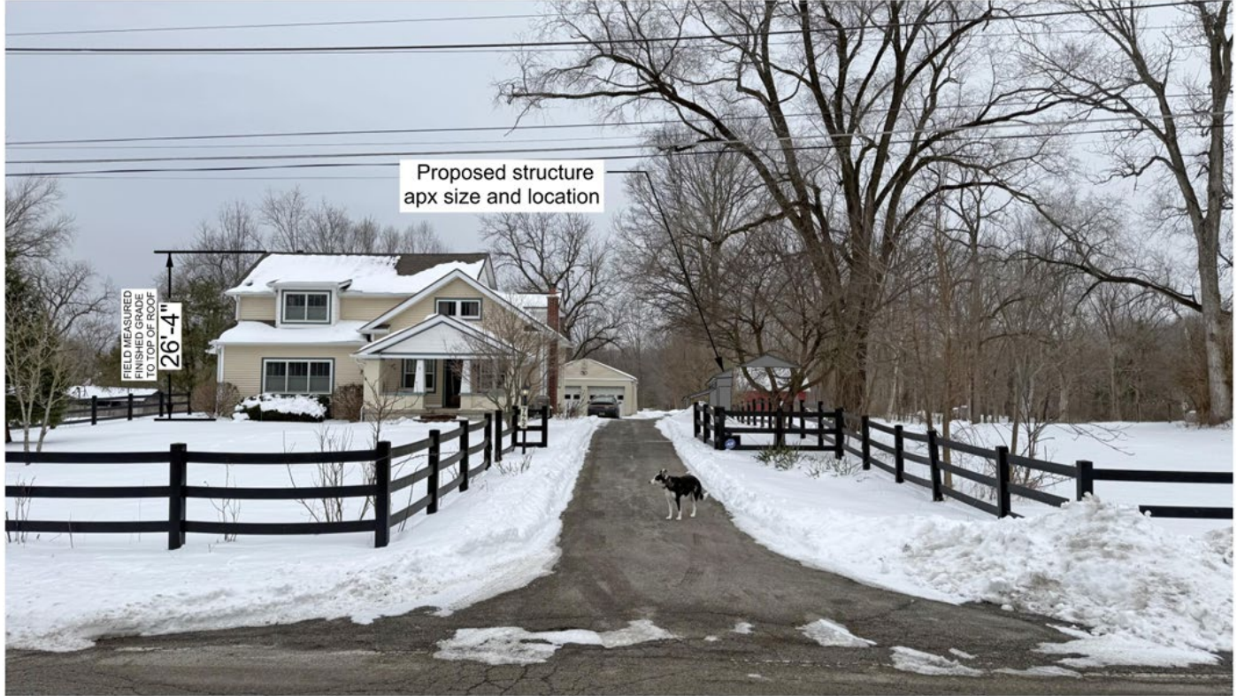
Property View From Street
