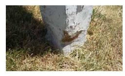
The damage to the wood post in the picture is from weed-eating around the base of the post. Over time, enough wood is lost that the post cannot take the weight of snow being pushed off the road. There are metal and plastic wooden post protectors that may be purchased to protect wooden posts from being weakened due to weed-eating. Lowe's has them for about \$8 and they install in seconds with no tools.
