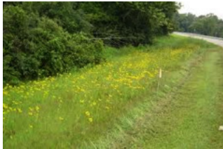
Example of Vegetated Filter Strip. Photo Credit: Wayne County Department of Public Services.
