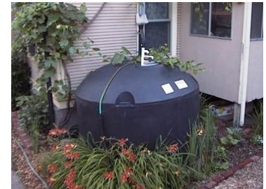
Example of above ground cistern
