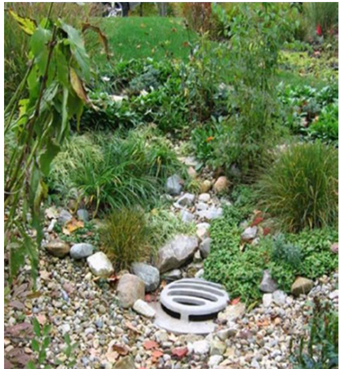
Example of rain garden with overflow structure.
