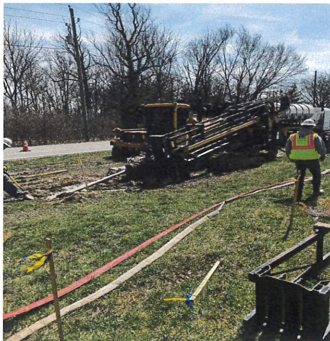
5400 Carroll Road - new HDPE pipe ready for installation and the Drill Rig
