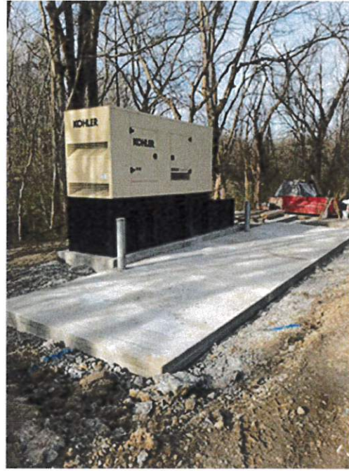
New emergency generator at IL WTP
