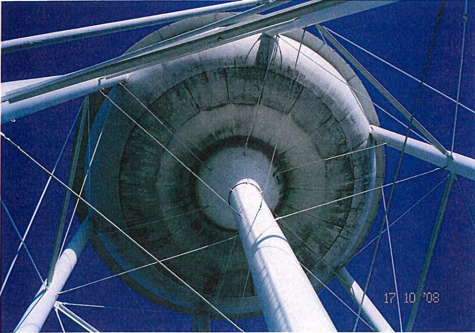
29. Bowl, riser, and riser rods. Note mildew on bowl.
