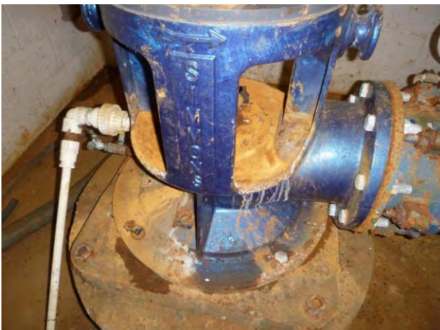
Well 14 Pump Head
