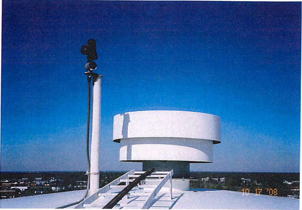
51. Obstruction light and roof vent.
