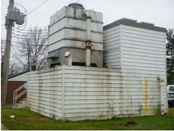
West Detention Tank
