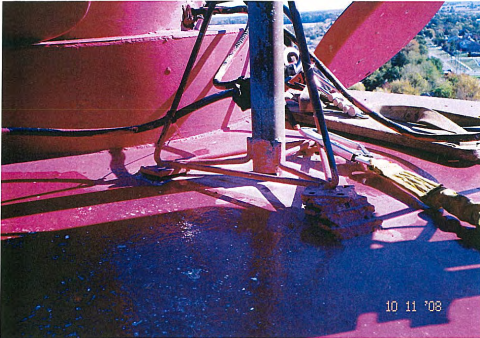
47. Antenna bracket on roof.
