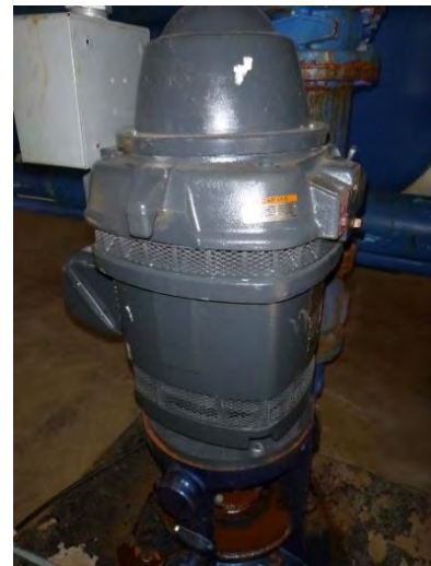
High Service Pump 3 Motor
