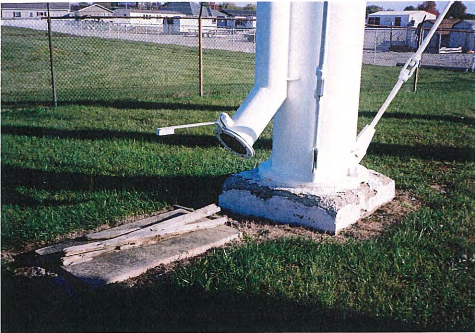
16. Discharge end of the overflow pipe.
