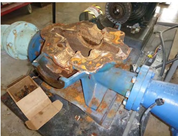
High Service Pump 3
