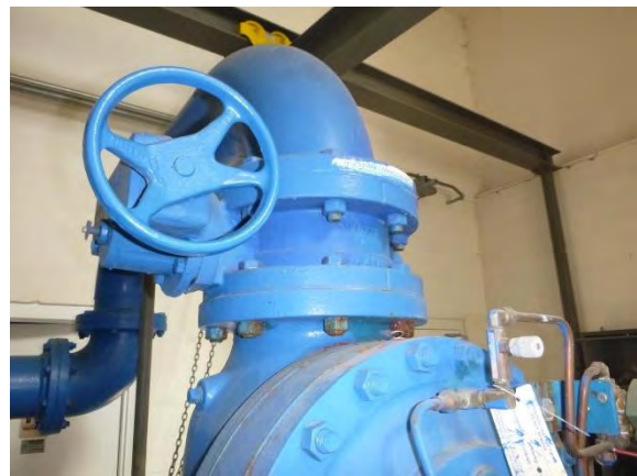
Manual Actuator in Pumping Building
