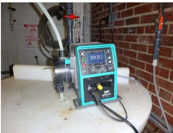
Pre-Filtration Chlorine Feed
