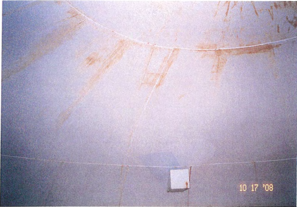
57. Interior roof and overflow weir box.
