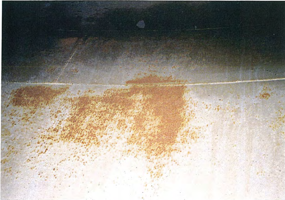
87. Corrosion on bowl.
