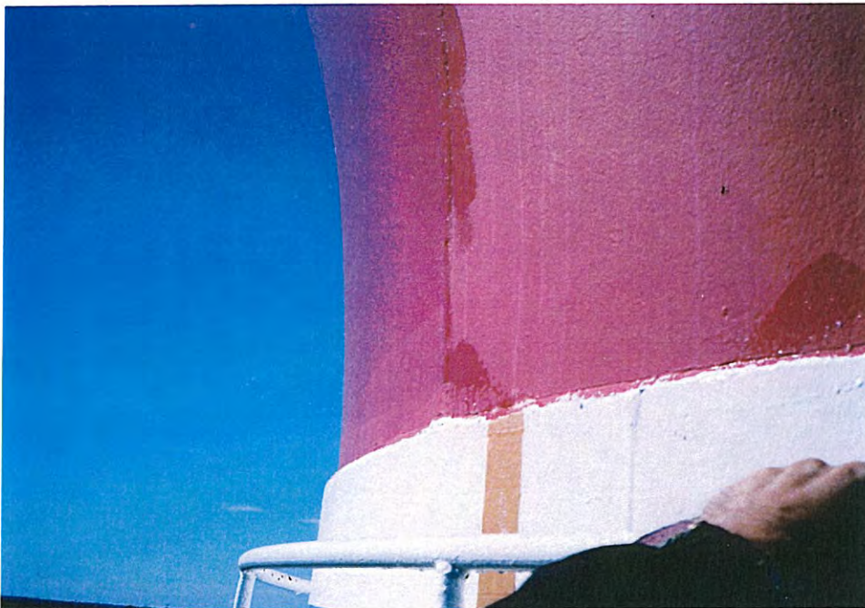
30. Faded coating on pedestal.
