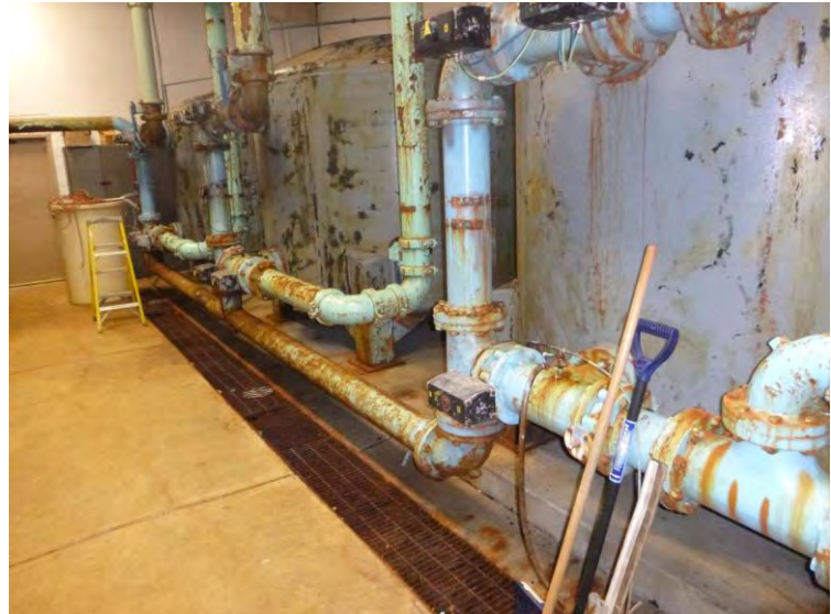
Corroded Process Piping
