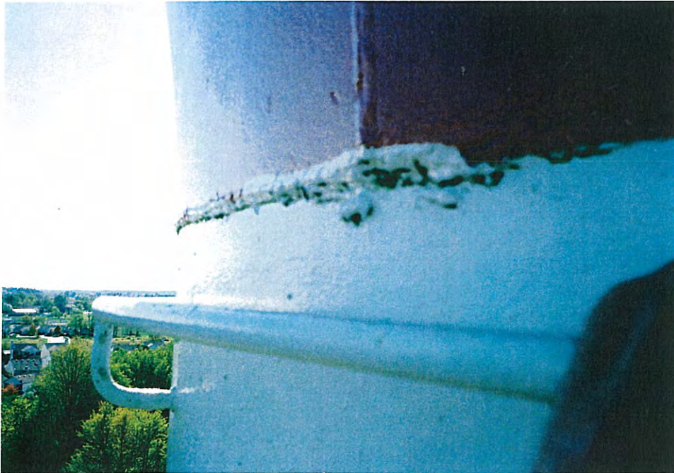
29. Painter's ring and mildew on pedestal seam.
