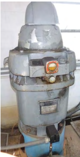
High Service Pump 2
