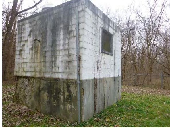
Well 10 Well House
