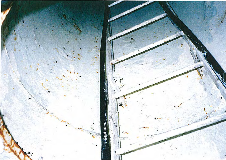
77. Access tube, ladder, and cables. Note corrosion.
