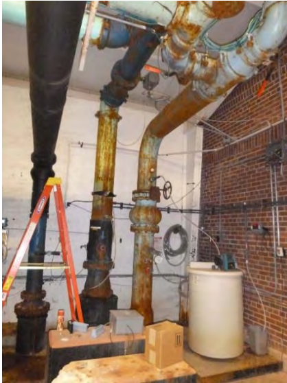
Process Piping & Chlorine Feed
