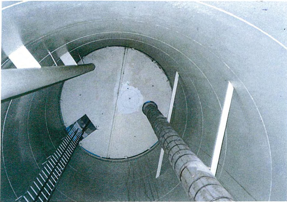
67. Pedestal, overflow pipe, inlet/outlet pipe, pedestal ladder, safe-climbing device, and underside of top platform.
