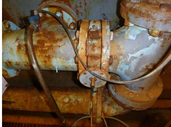
Butterfly Valve in Filter Building
