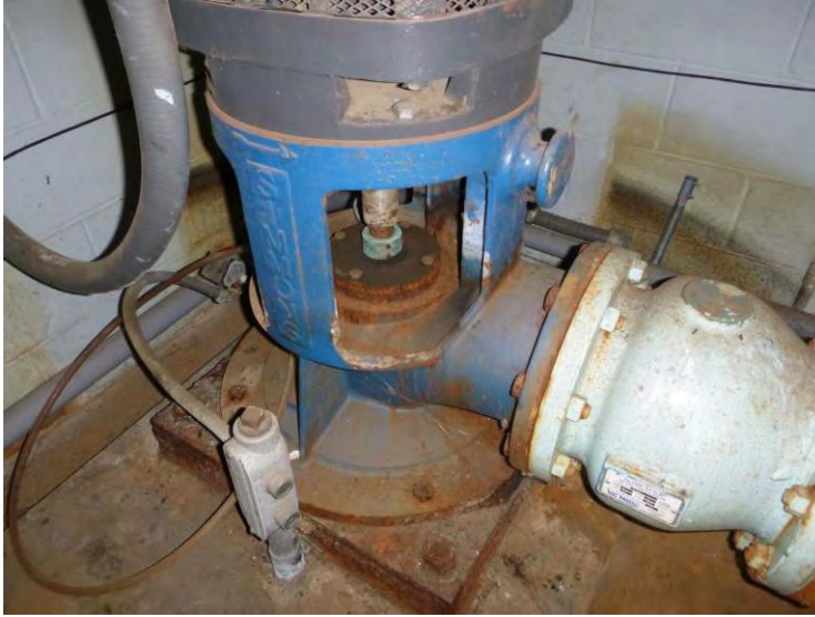
High Service Pump 3
