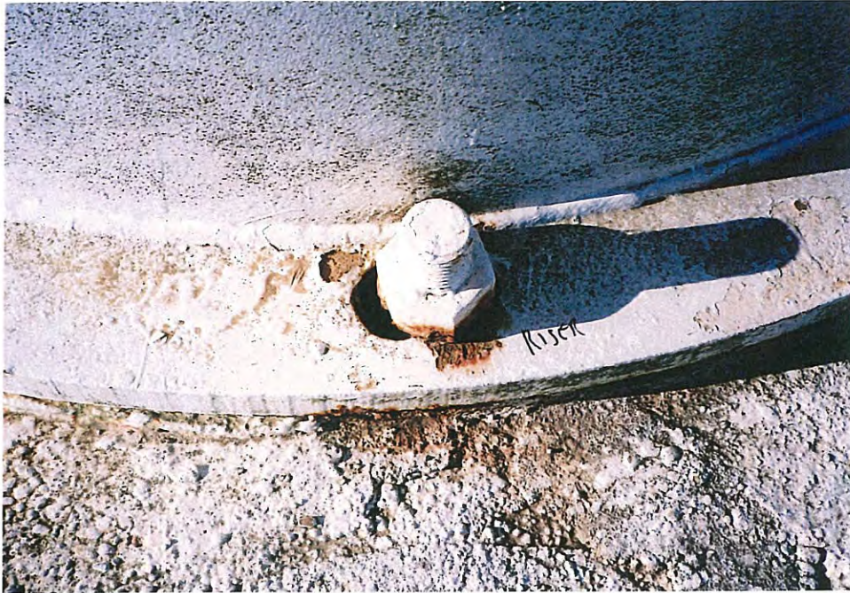
11. Riser base plate and anchor bolt. Note corrosion and gap at bolt hole.
