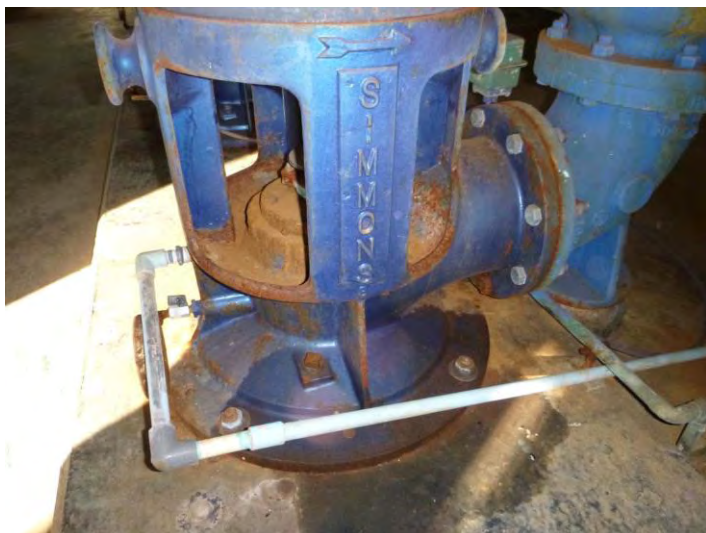
High Service Pump Head 1
