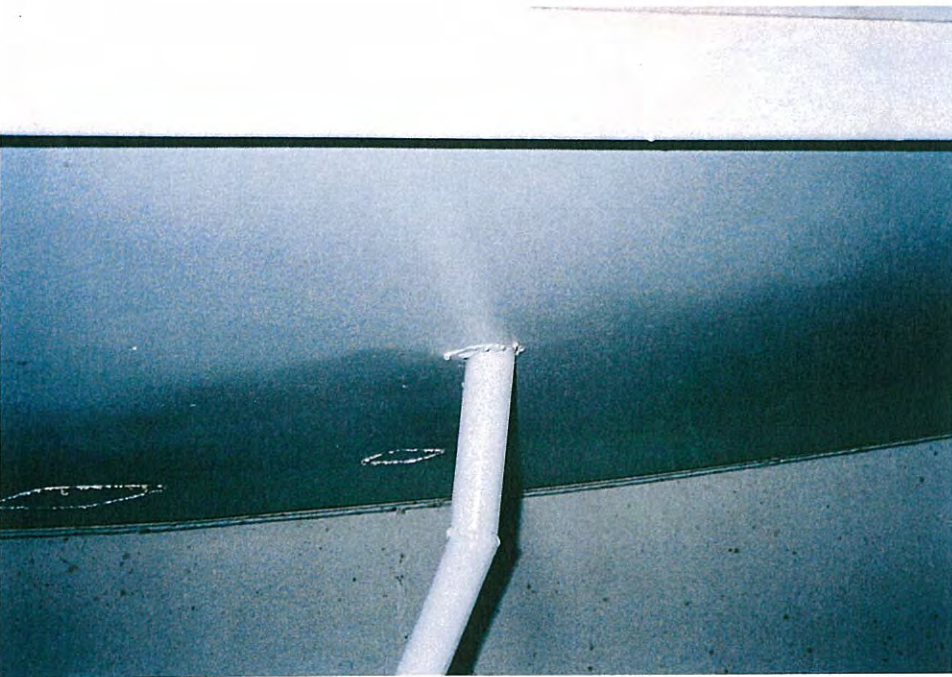
62. Condensate platform drain pipe.
