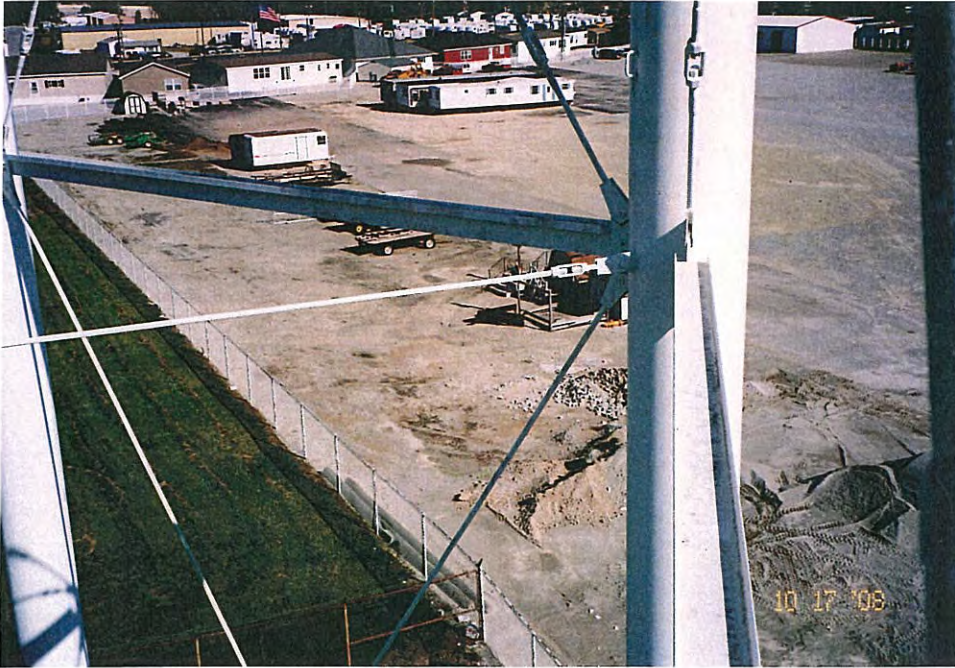
25. Column, struts, diagonal bracing, and riser rod.
