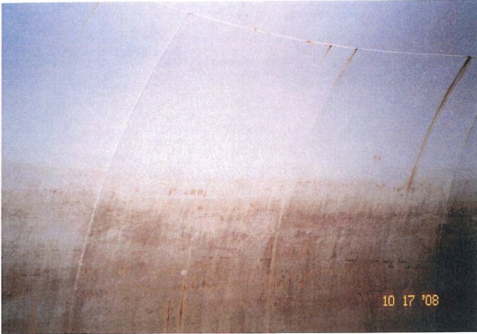
59. Interior roof knuckle.
