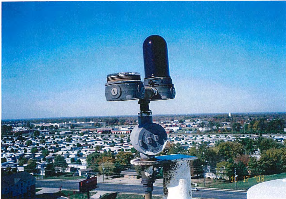
50. Obstruction light on roof. Note bulb and globe missing.
