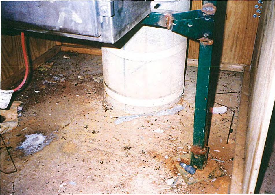
51. Dirt on base cone enclosure floor around inlet/outlet pipe penetration through concrete floor/
