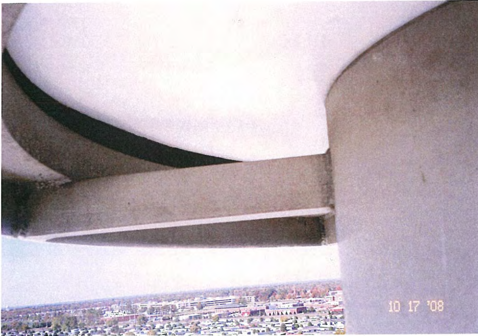
53. Gap at roof vent pallet.
