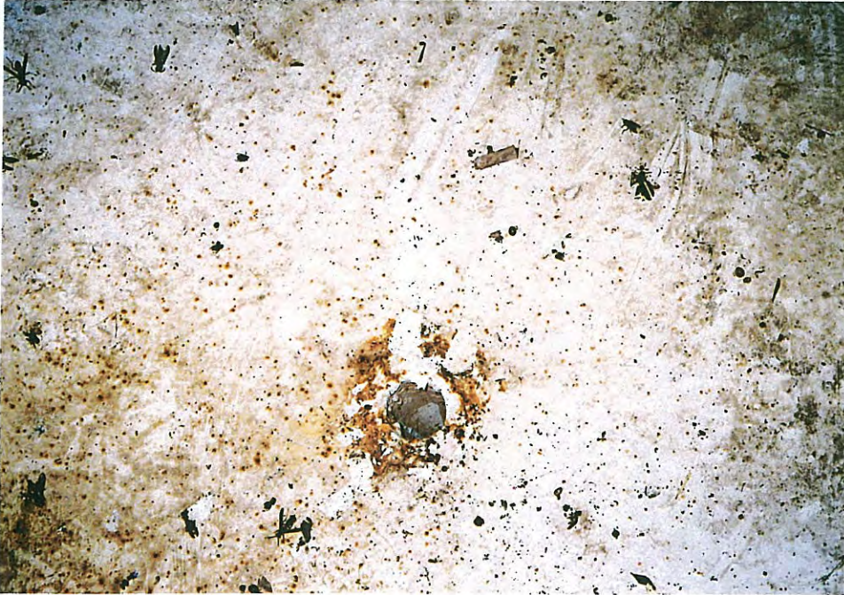
65. Dirt and corrosion around drain hole in condensate platform.
