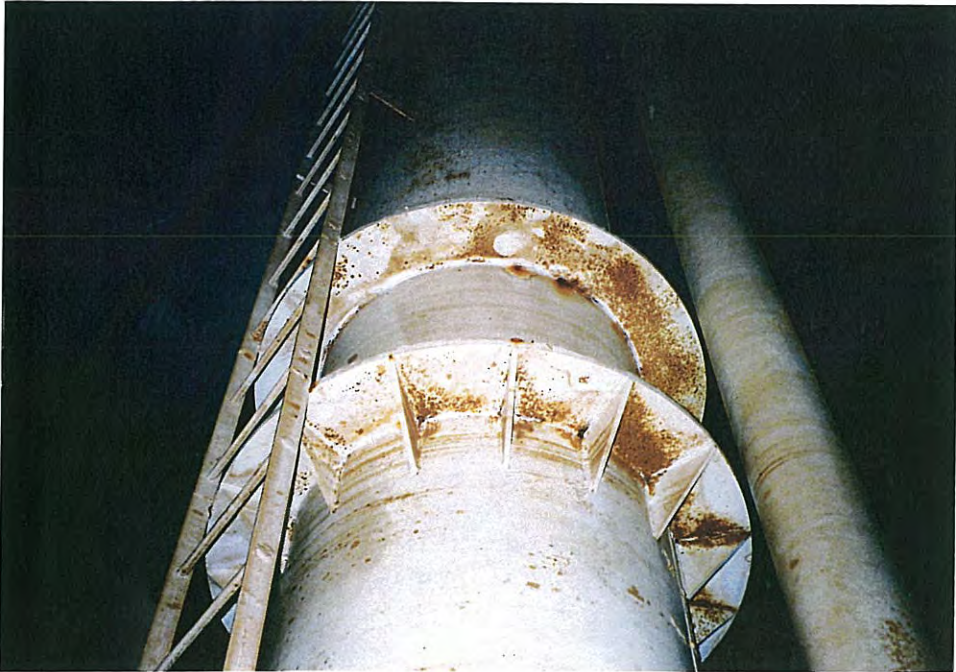
91. Wet ladder and access tube stiffeners.
