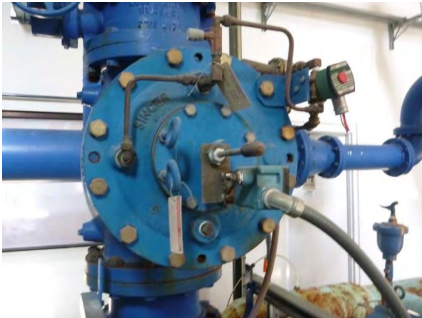
Process Piping in Pumping Building
