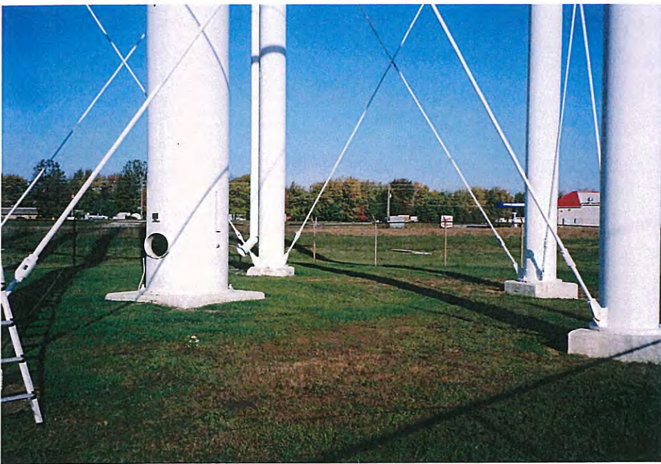
12. Columns and riser.
