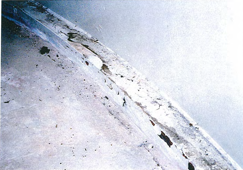
53. Peeled coating on interior dry base plate projection.
