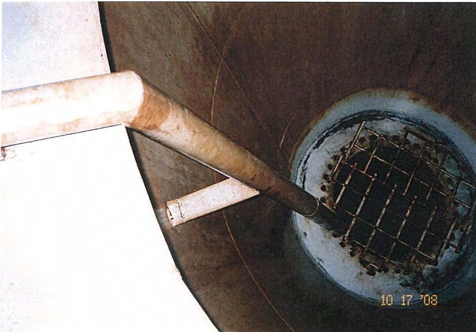
68. Siphon pipe in transition cone.
