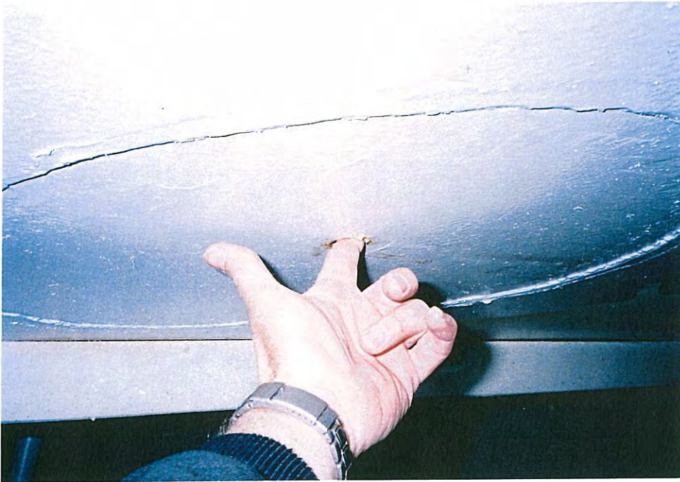
61. Hole in condensate platform.
