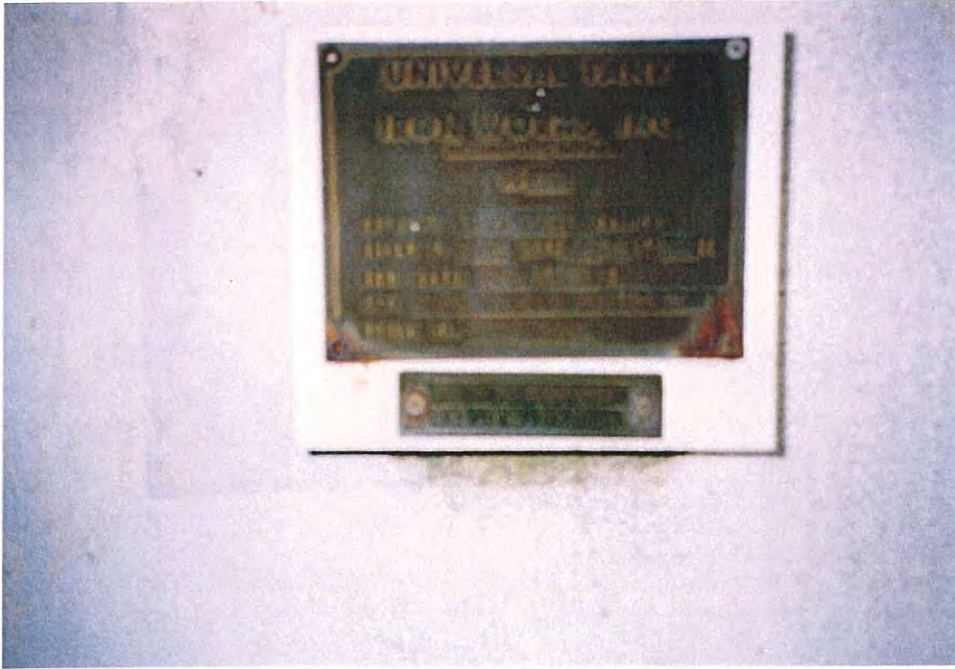
15. Tank nameplates on riser.
