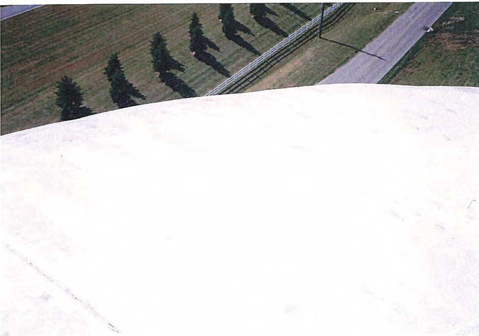
48. Weathered topcoat on roof.
