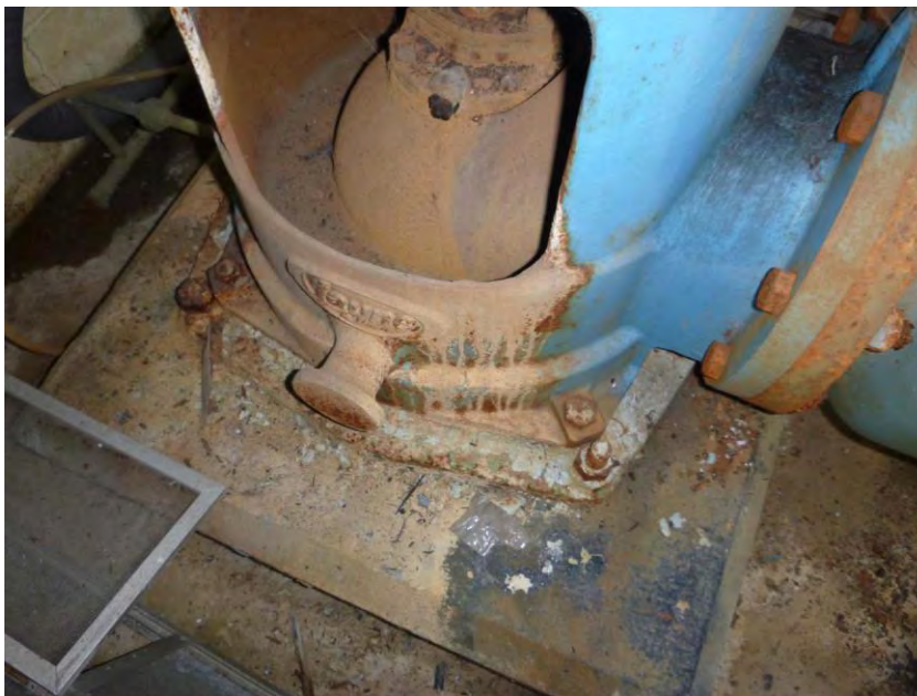
High Service Pump 2
