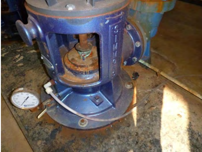
High Service Pump 2
