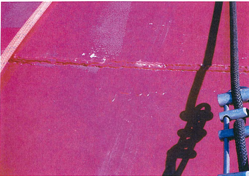
38. Faded graphic coating on roof.
