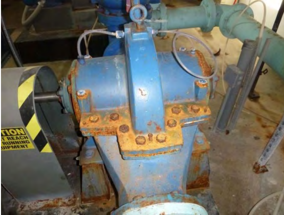
High Service Pump 2
