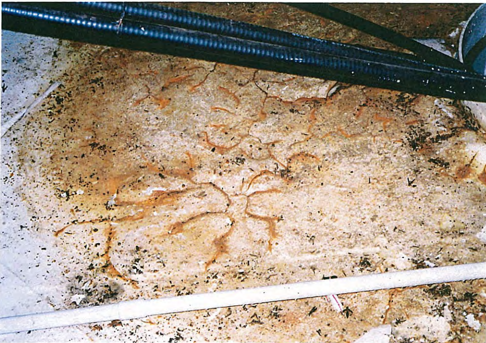
64. Evidence of accumulated water on condensate platform. Note failed coating.
