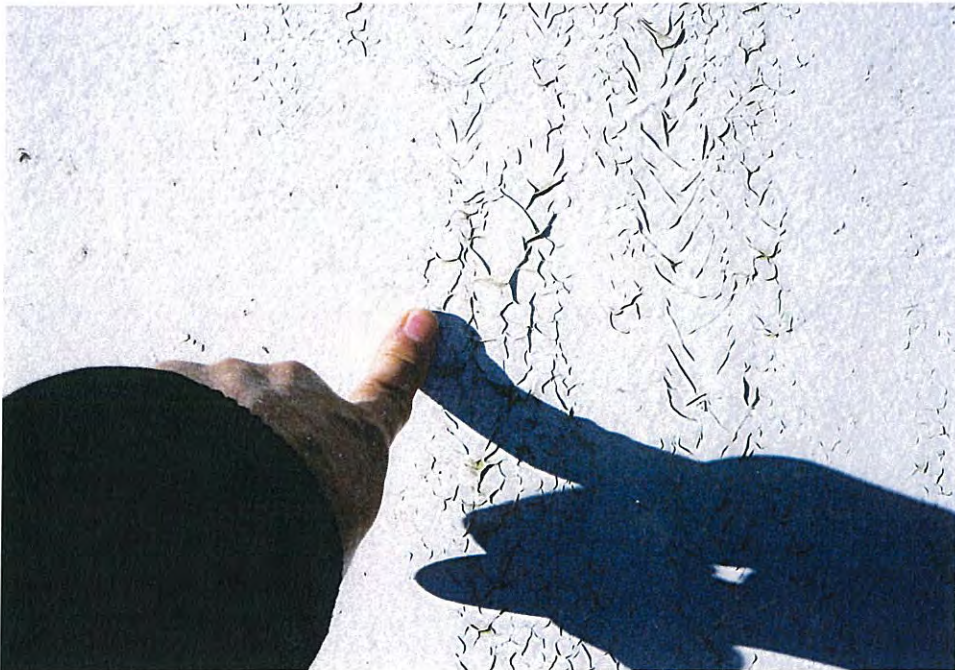
22. Cracked base cone coating.
