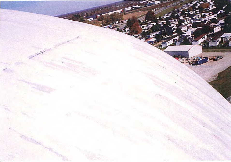
47. Weathered topcoat on roof knuckle.
