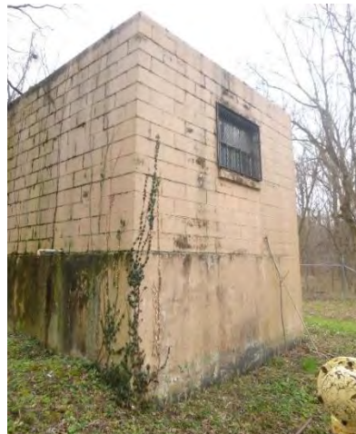
Well 9 Well House
