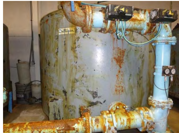
Process Piping in Filter Building
