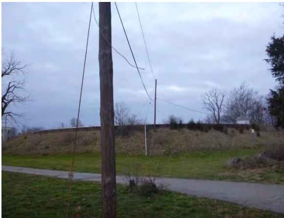
3 MG Ground Storage Reservoir
