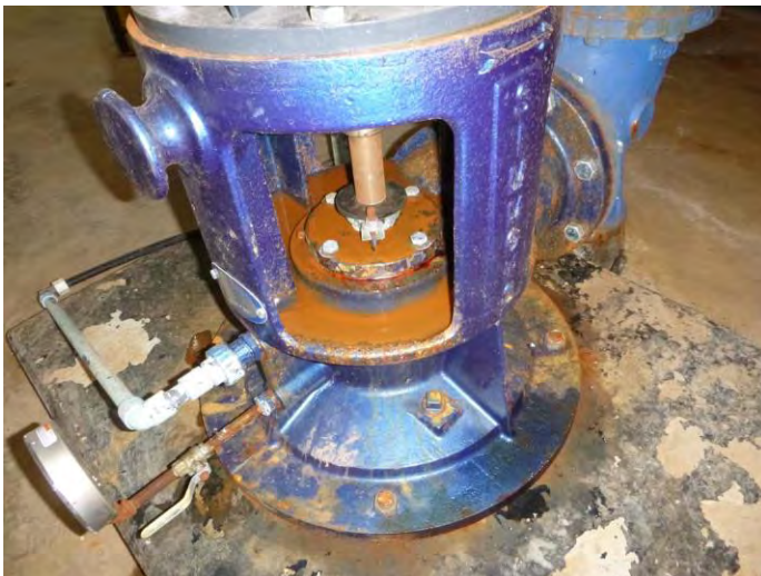
High Service Pump 3
