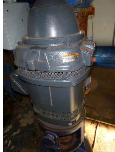
High Service Pump 2 Motor
