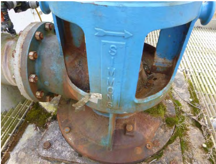
Well 8 Pump Head
