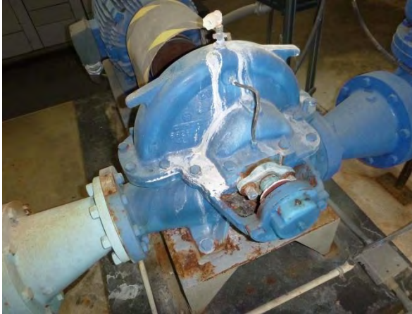
High Service Pump 1
