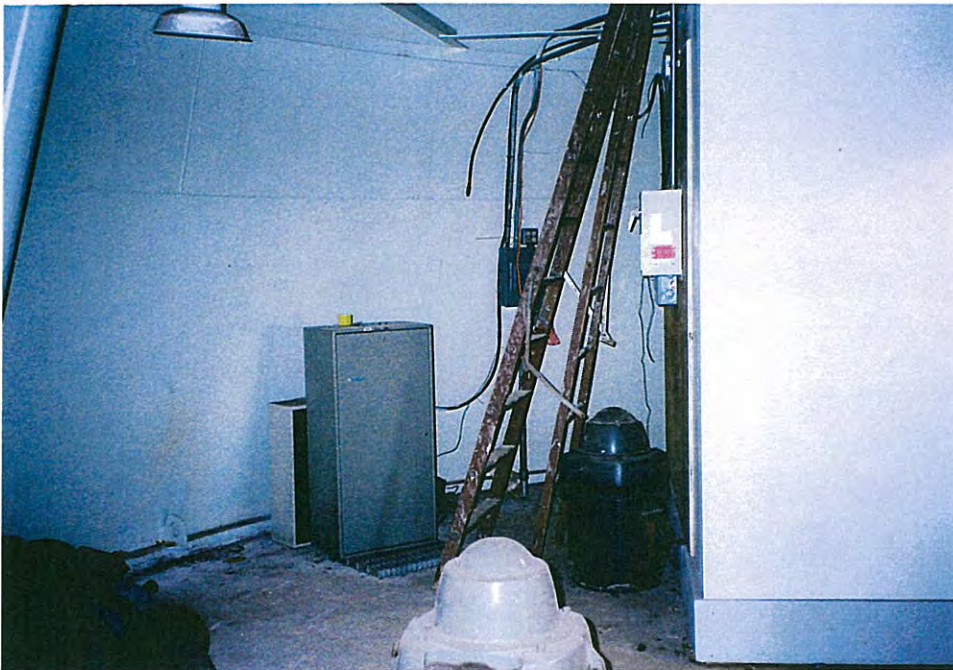
52. Electrical cabinets and unused pumps in base cone.
