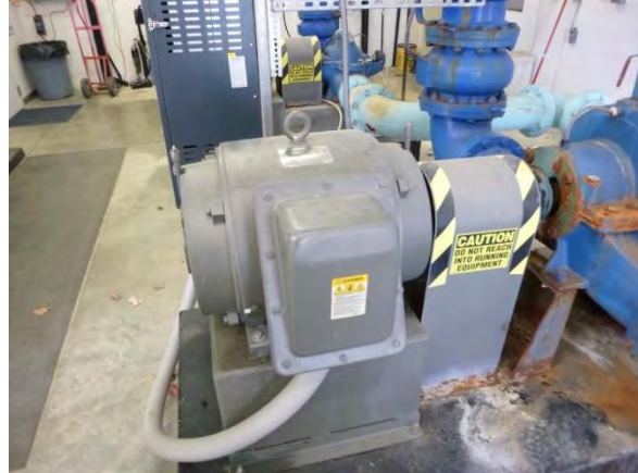
High Service Pump 2 Motor
