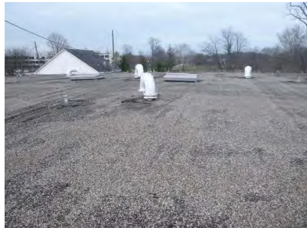
3 MG Ground Storage Reservoir Roof
