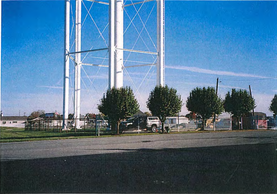
5. Tank and site.
