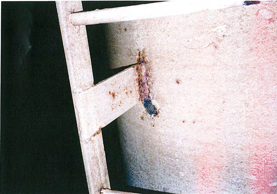
92. Corrosion on wet ladder bracket.
