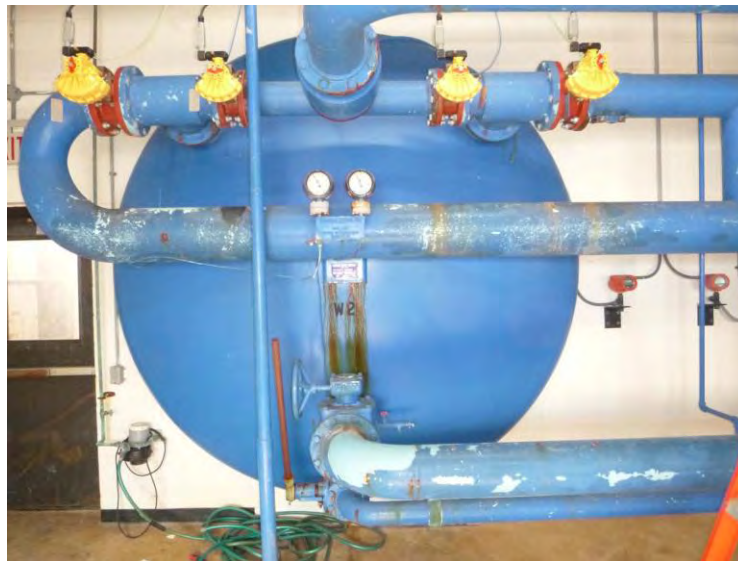
Filter W2, Process Piping, Valves, and Actuators
