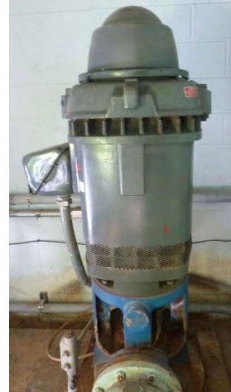
High Service Pump 4
