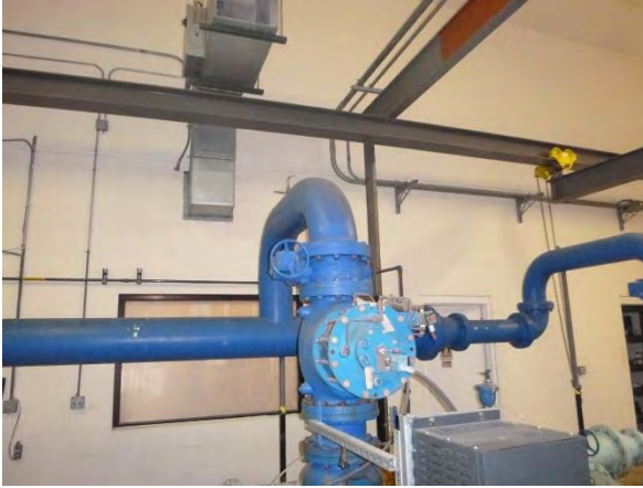
Butterfly and Check Valve in Pumping Building
