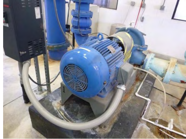
High Service Pump 1 Motor
