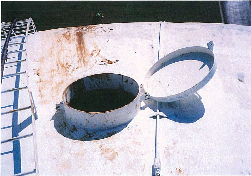
49. Roof manhole and ladder.
