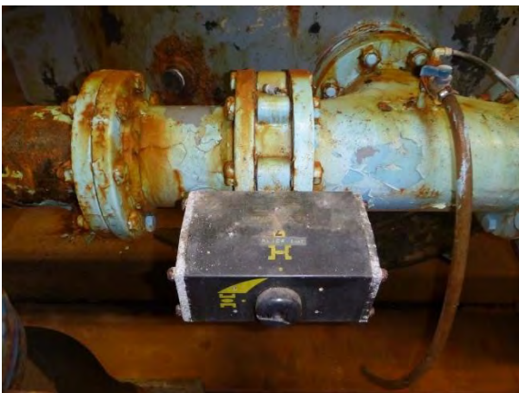
Electric Actuator in Filter Building
