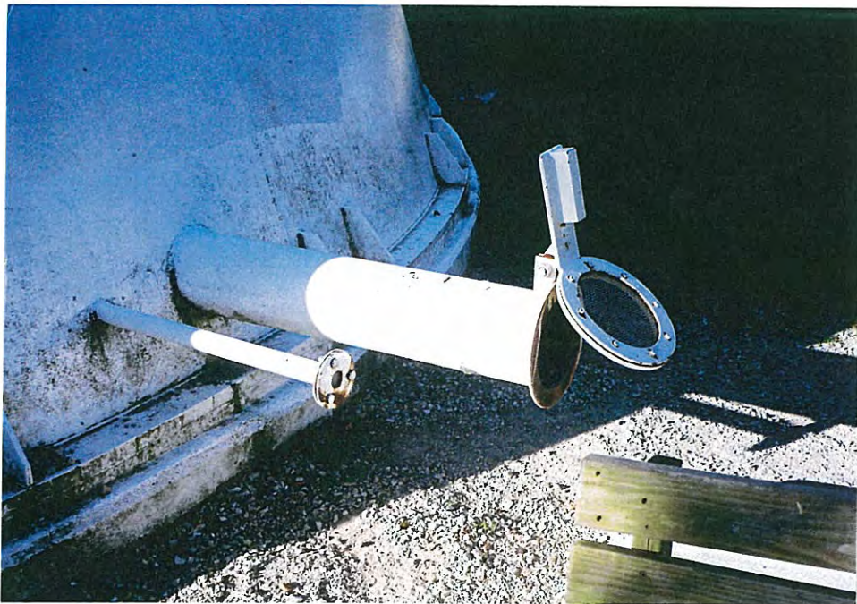
12. Overflow pipe and condensate pipe discharges.
