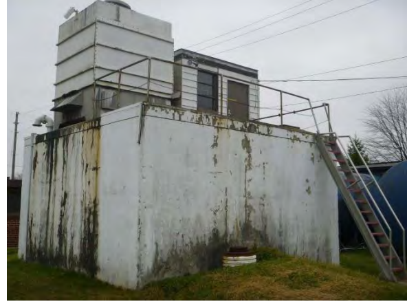
East Detention Tank
