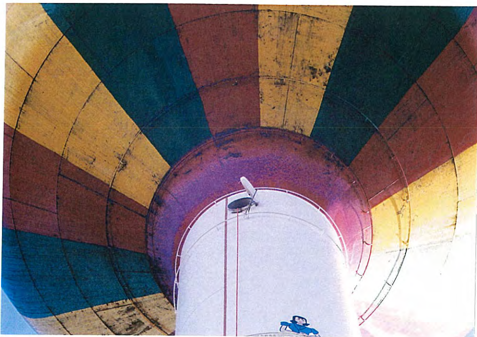
27. Painter's rings and painter's manhole.
