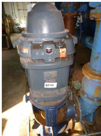
High Service Pump 1 Motor
