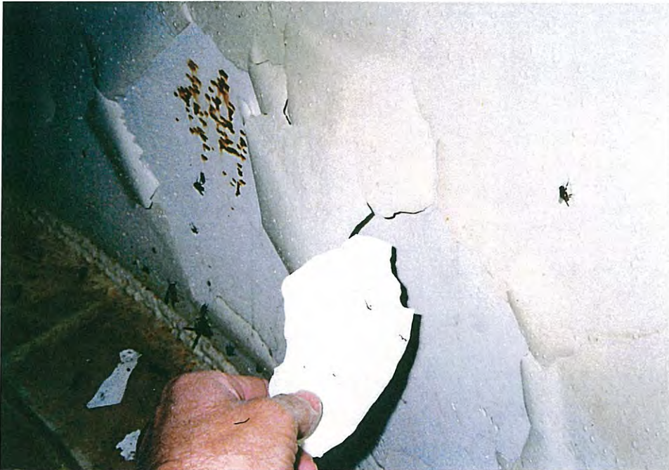
66. Peeled topcoating and corrosion on pedestal just above condensate platform.
