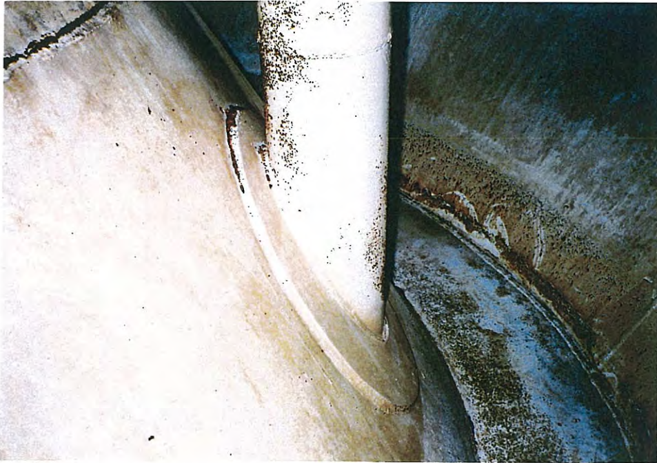
95. Overflow pipe penetration through bowl cone.
