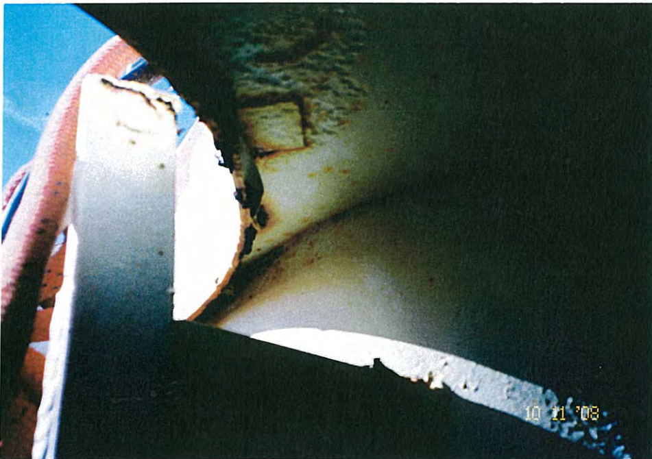
78. Corrosion around access tube penetration through wet roof.
