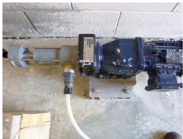
Post-Filtration Chlorine Feed
