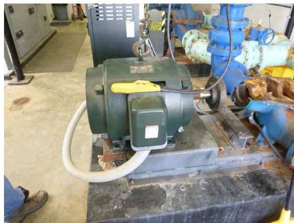
High Service Pump 3 Motor
