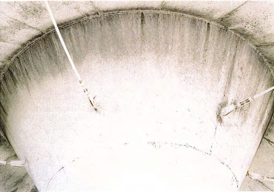
30. Riser rods and transition cone below bowl.
