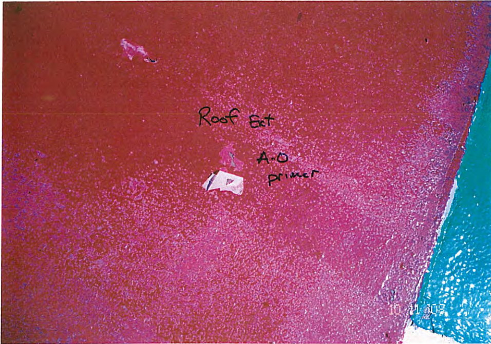
41. Coating adhesion test on roof.
