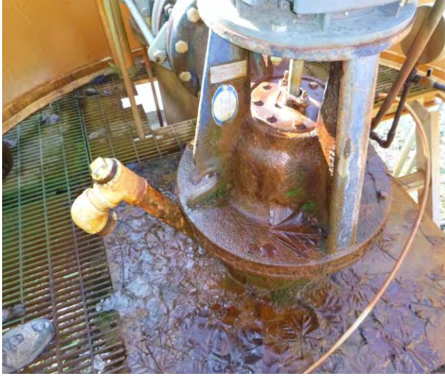
Well 15R Pump Head
