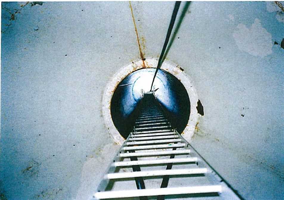
76. Dry bowl, access tube, and ladder.
