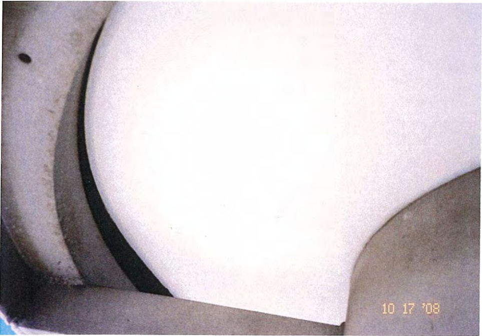
52. Gap at roof vent pallet.
