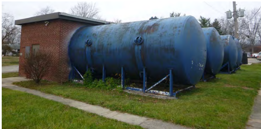
Horizontal Pressure Filters
