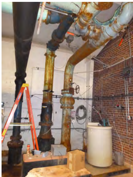
Process Piping & Chlorine Feed
