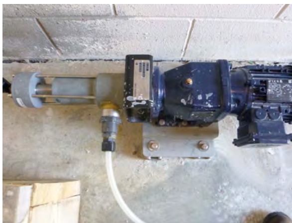
Post-Filtration Chlorine Feed
