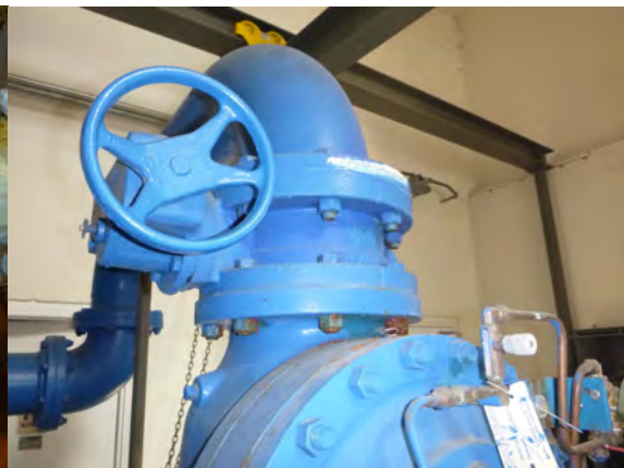
Manual Actuator in Pumping Building
