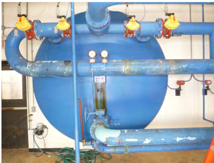
Filter W2, Process Piping, Valves, and Actuators
