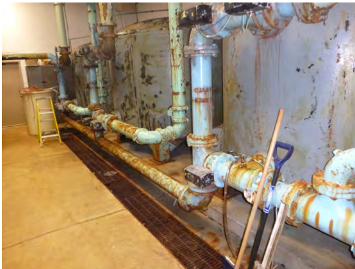
Corroded Process Piping
