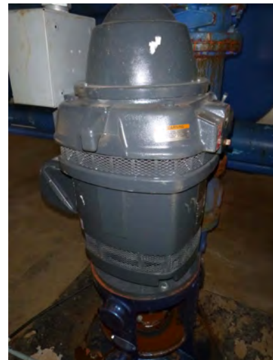
High Service Pump 3 Motor
