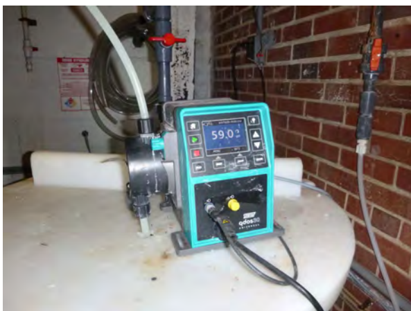
Pre-Filtration Chlorine Feed
