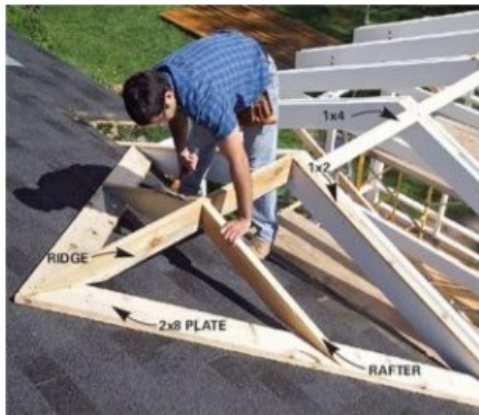
The new roof extends onto an existing roof using a ridge board. No loads from the new roof are transferred to the existing dwelling. The existing roofing has not yet been trimmed.
