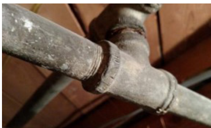
Galvanized Pipes
