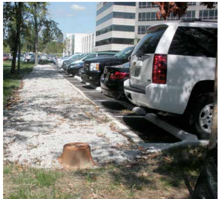
An infiltration trench to capture parking lot runoff. Subsurface access is shown in the foreground.
